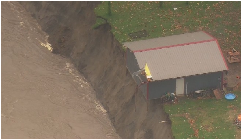
Lyman – 80 Feet of Bank Erosion
