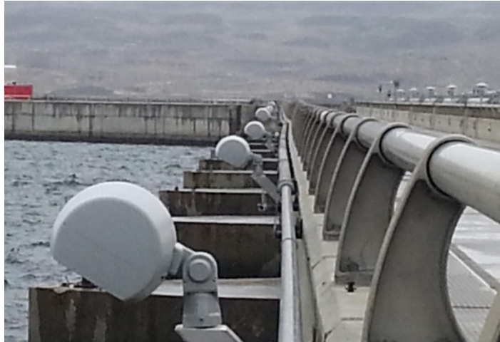
Deflection visible at the top of Wanapum Dam (PUD #1)
